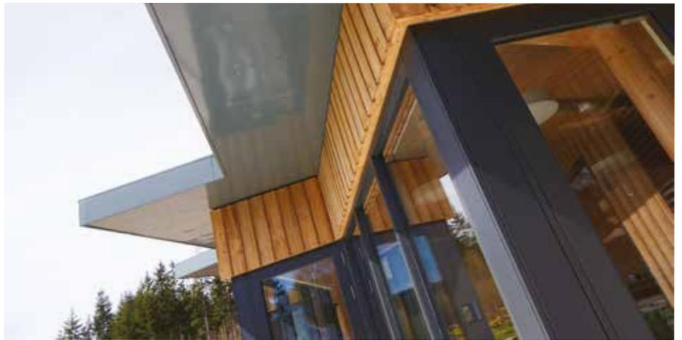
timber panels form the spine wall and roof deck, supported on glulam beams and columns. To speed up construction, contractor William Gray Construction prefabricated the external timber frame offsite. The Scotlarch was finished with a SiOO:X treatment, ensuring the timber will weather at an enhanced rate and settle into its surroundings.
